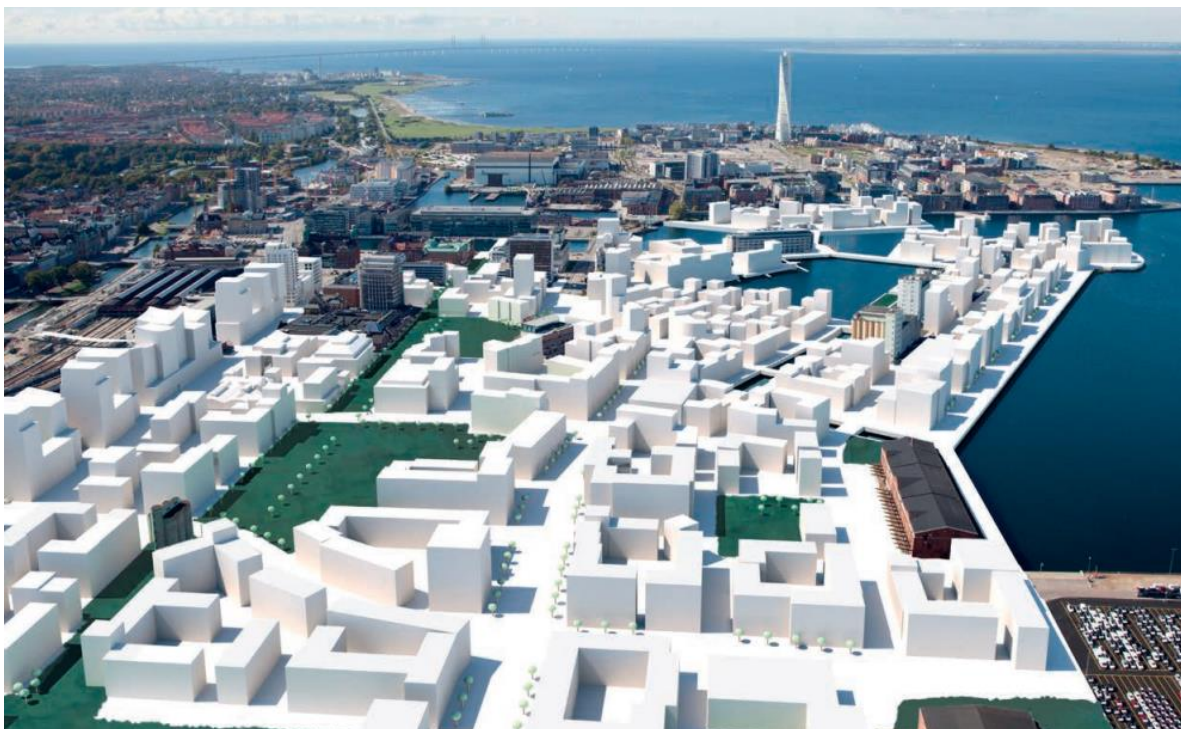
Figure 1: Planned Nyhamnen extension, with Bo01 neighbourhood in the background (Image: Malmö stad, 2019)
