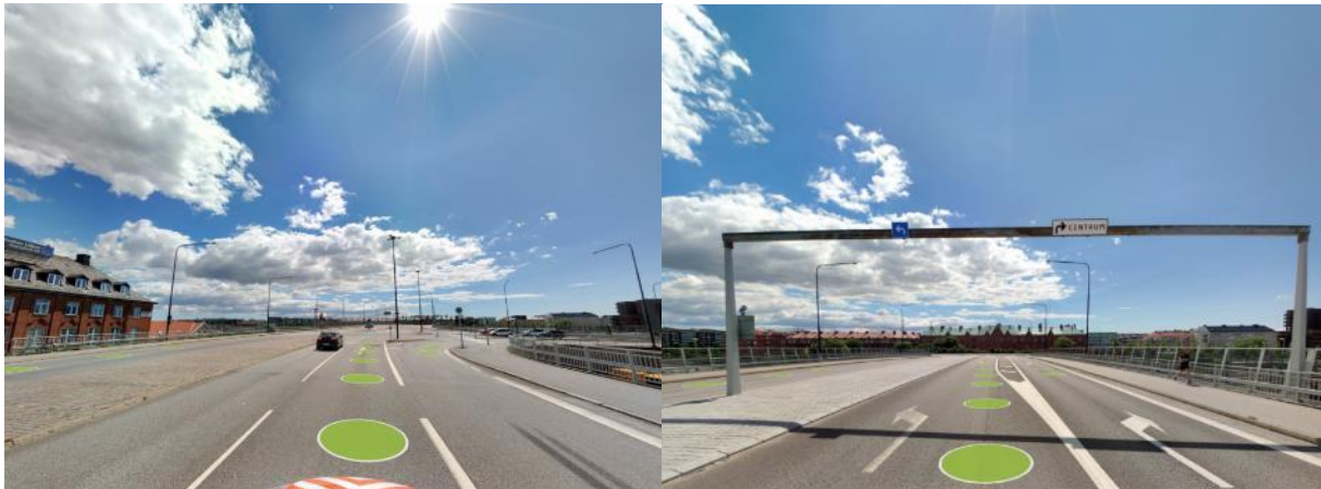
Figure 85. Frihamnsviadukten (segment 5), to the south
