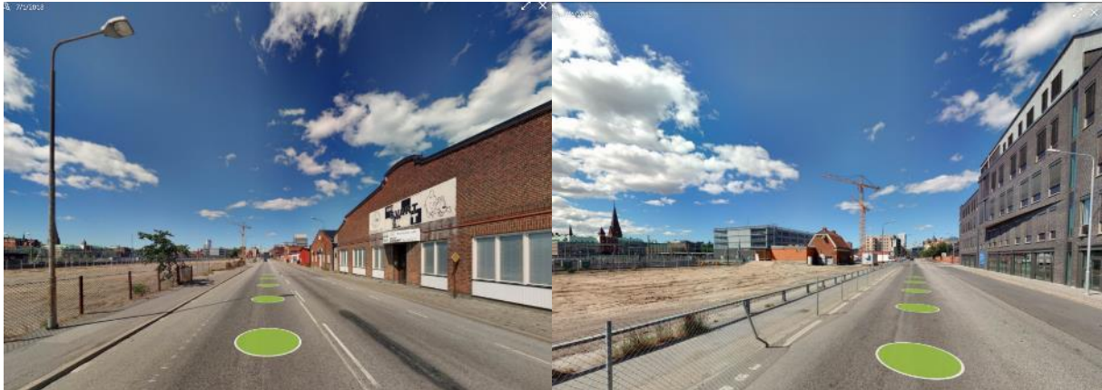
Figure 88. Carlsgatan (segment 8), looking west
