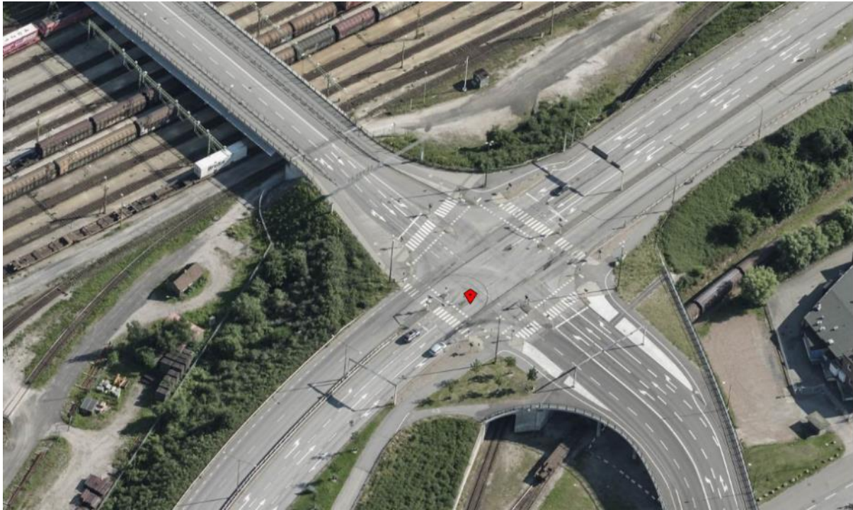
Figure 82. Sjölundaviadukten overview, looking south-west
